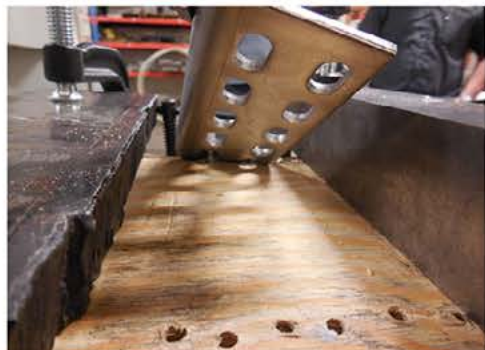
Photo 4: Closeup of Fastener Pullout & Failure
