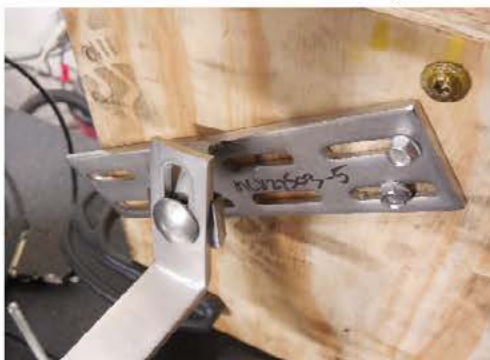
Photo 12: Typical Failure Mode - Deformation at Weld
