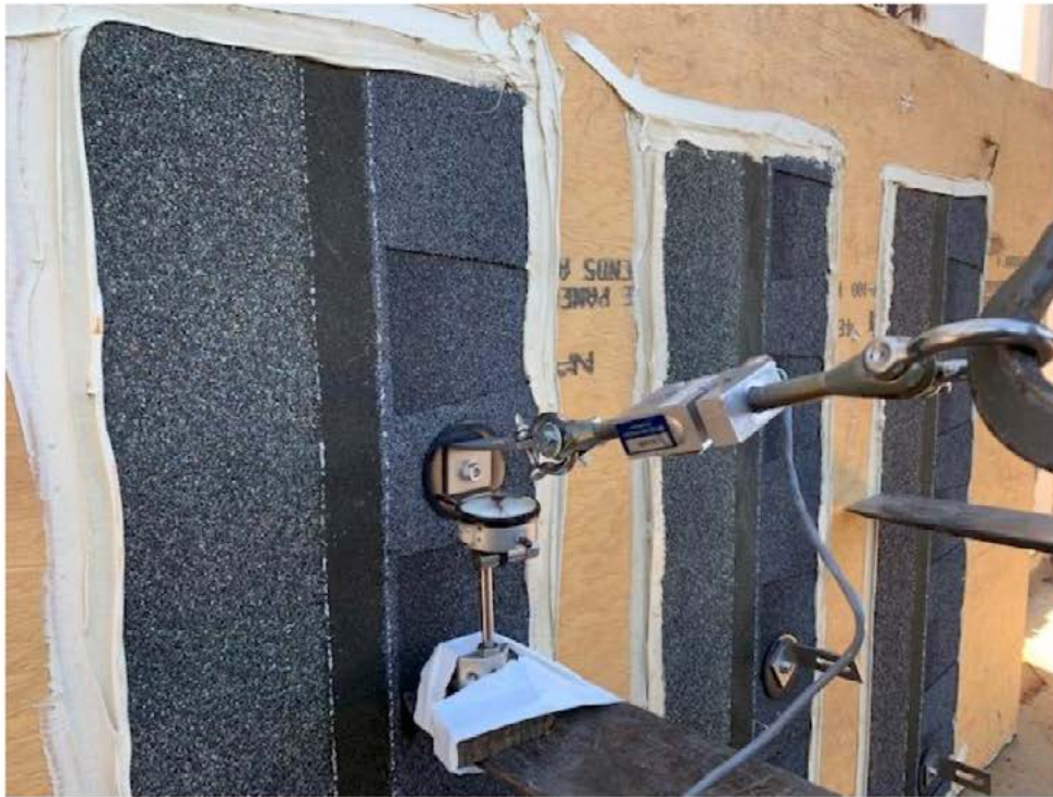
Photo No. 1 Pullout Test
