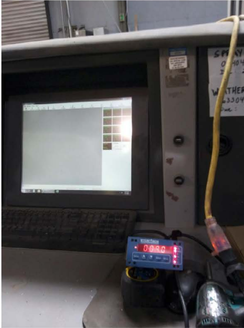
Photo No. 5 Instrumentation
